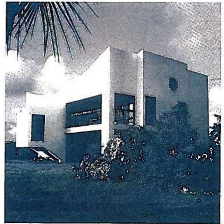
DEAL RESIDENCE-PARTIALLY AIR CONDITIONED SUNSET PORCH, LEeward SIDE
